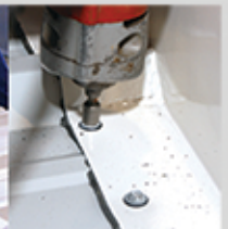
Secure Roof Curb into place using Self-Drilling screws
