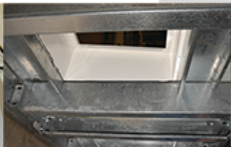
Install the necessary framework around the hole
